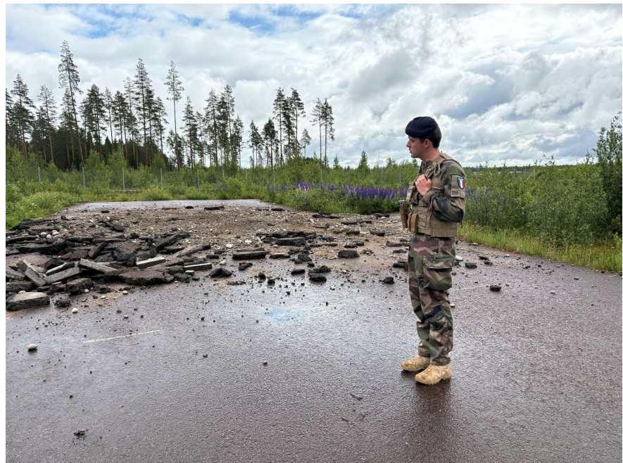
Figure 33: Dedicated units able to repair combat damage to transport infrastructure are a key capability, although sometimes an overlooked one. Due to the nature of transport infrastructure, realistic training opportunities can sometimes be difficult to find, but here the French Air and Space Forces' 25e régiment du génie de l'air (25 RGA, the 25th engineering regiment) has gotten the opportunity to repair holes blown in the tarmac of Halli airport. Credit: Robin Häggblom/Risk Intelligence A/S
